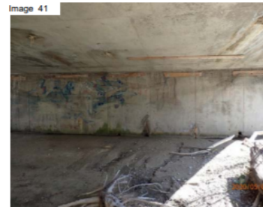
East abutment wall
