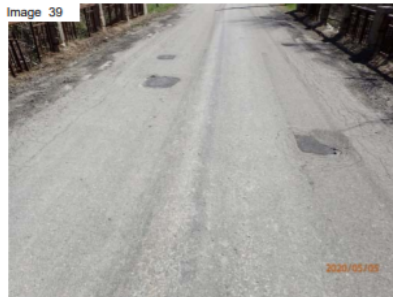
Asphalt on deck
