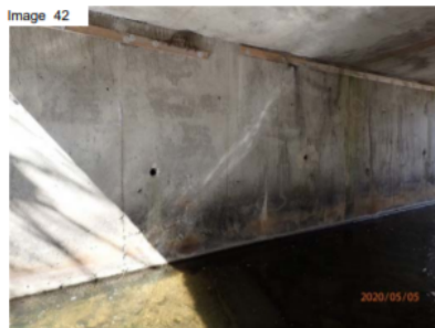
West abutment wall
