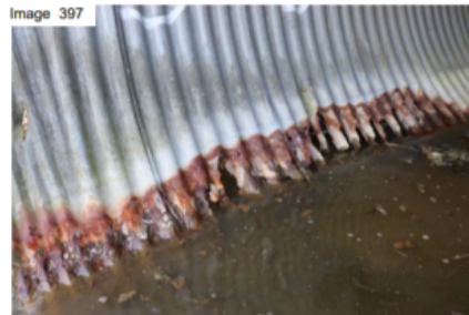
North inlet perforation
