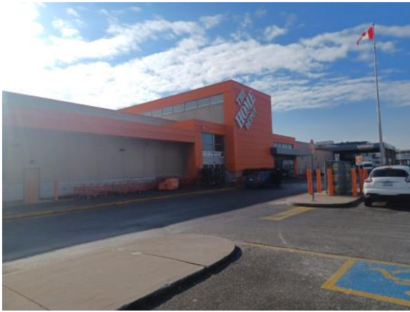
Photo 1: View of the north wall of the Site building occupied by Home Depot. Photograph taken facing southwest.
