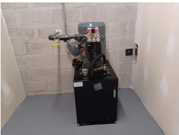
Photo 11: View of the hydraulic unit for the freight elevator for Shoppers Drug Mart at 1105 D Kingston.
