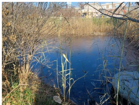
Photo 12: View of the storm water management to the northwest of the Site building occupied by Michaels.
