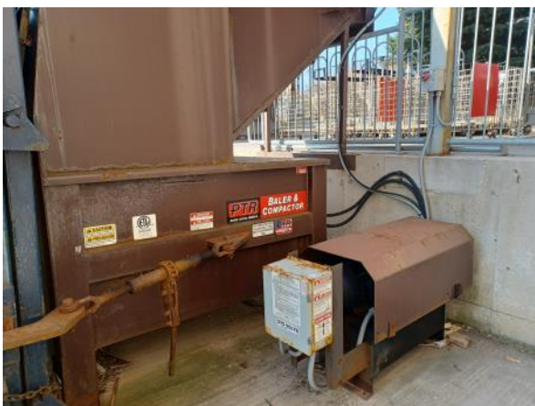
Photo 11: View of the hydraulic oil operated garbage compactor west exterior to the Site building occupied by Michaels.
