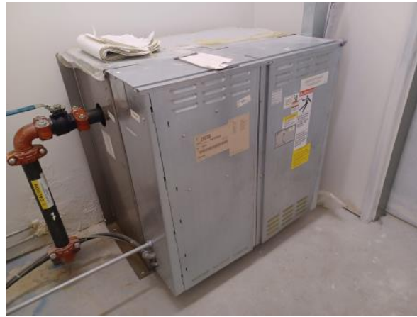
Photo 8: View of the hydraulic unit for the passenger elevator for the second floor commercial units at 1105 E Kingston Road.
