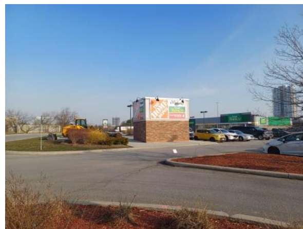
Photo 6: View of the water building in close proximity to the north Site boundary.
