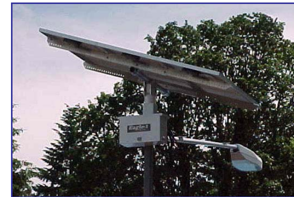
Solar powered light standard
