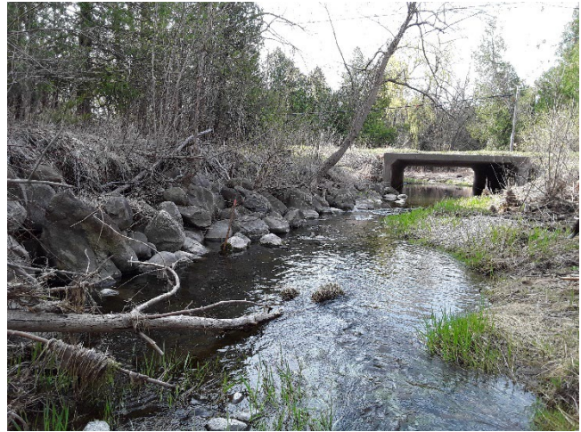
Photograph 2. Location 2. Reach PC-1 Petticoat Creek.
