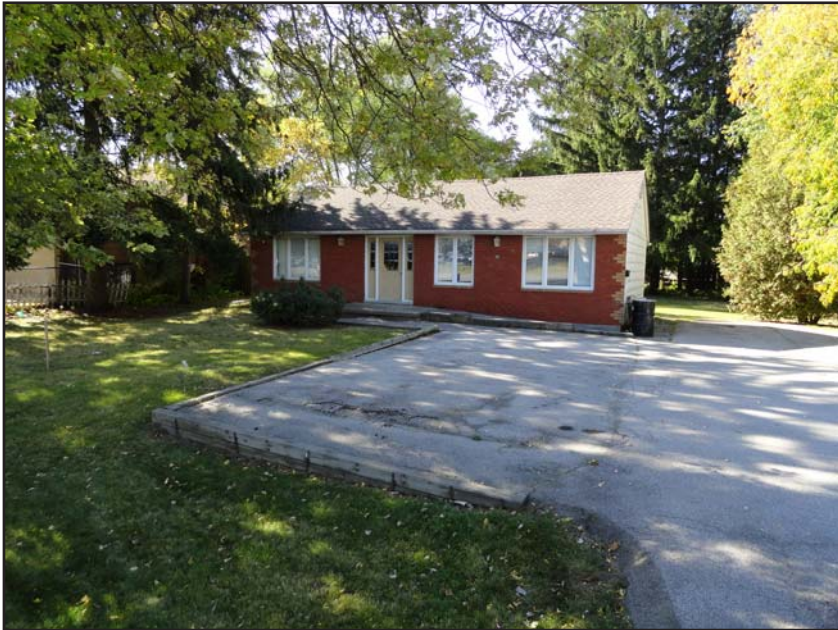
Photograph 13. View of front of 1 storey single-family dwelling at 1854 Liverpool Road (part of CVR_3 )
