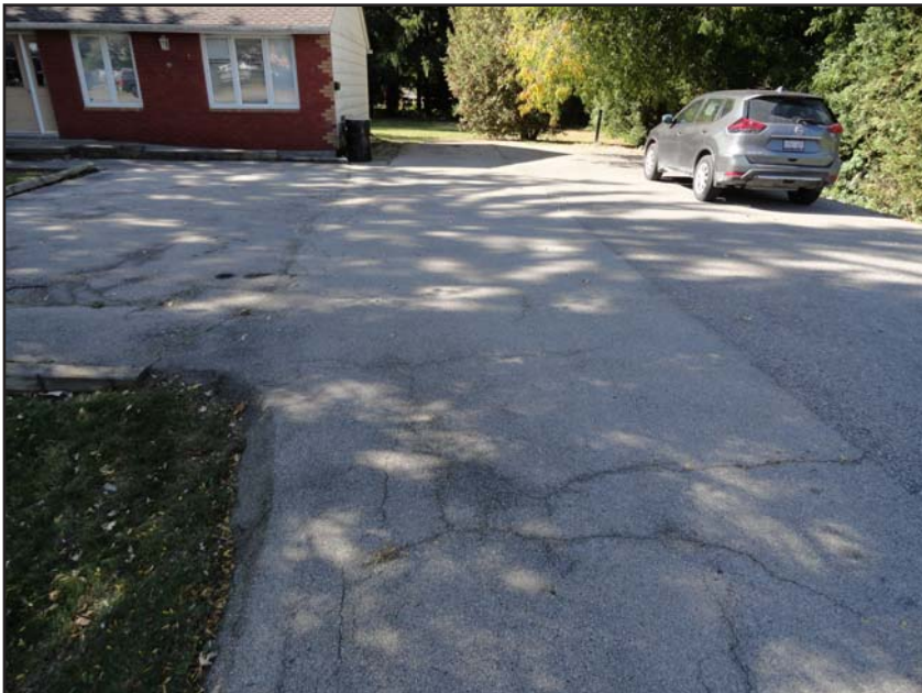
Photograph 3. View westward of driveway at 1854 Liverpool Road
