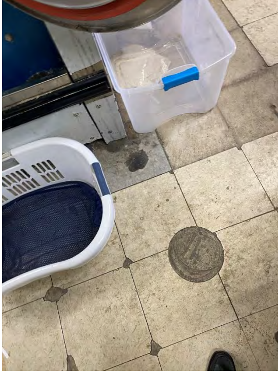
Photo 3: Dry Cleaners. View of Floor.
