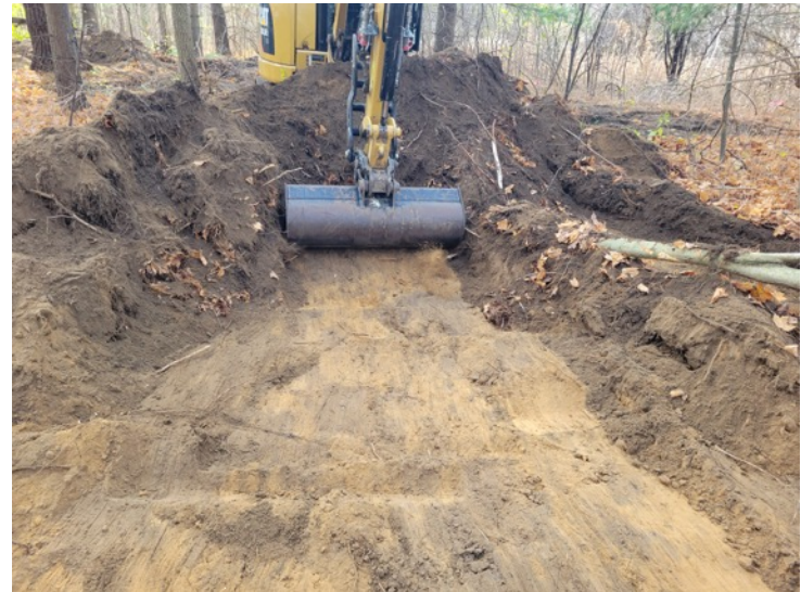
Image 12: MTR in progress at the west part of the site.
