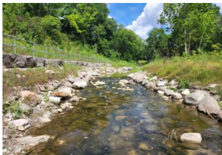
An example of natural channel design enhanced with vegetated buttress
