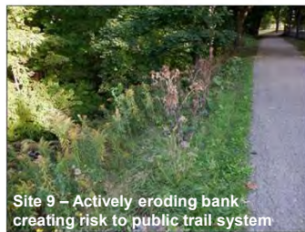
Site 9 – Actively eroding bank creating risk to public trail system
