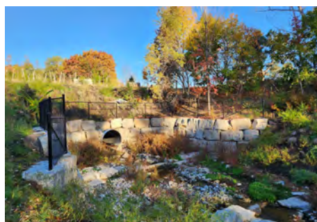
An example of culvert rehabilitation and downstream scour pool works
