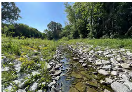
An example of a stone lined drainage channel
