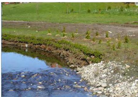
An example of natural channel design enhanced with vegetated butress
