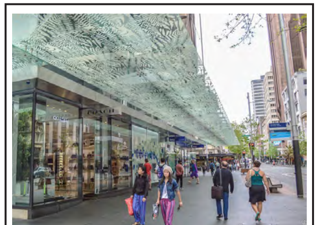
Use of awnings to provide weather protection
