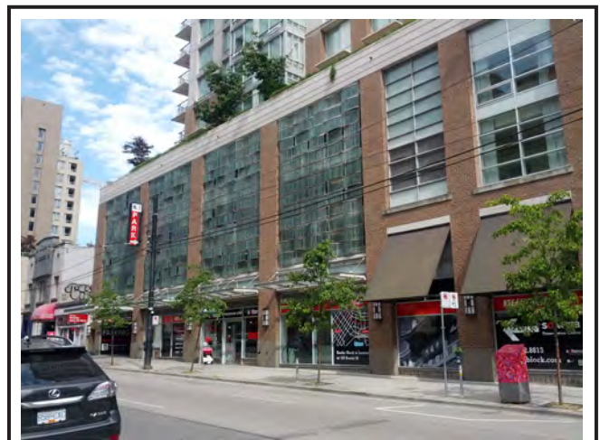
Structural above grade parking with active uses at grade
