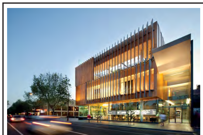
Public buildings should be characterized by high quality architectural design
