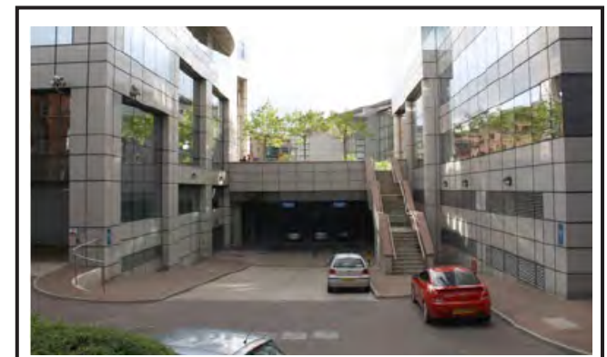
Underground loading and unloading
