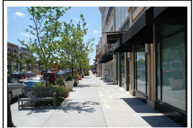
Buildings aligned to create a consistent street wall
