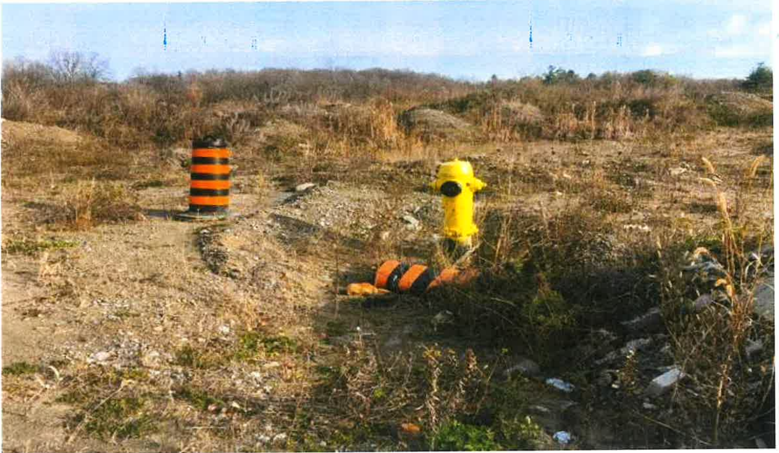
General view of fire hydrant in southwest portion of the subject site (looking east).
