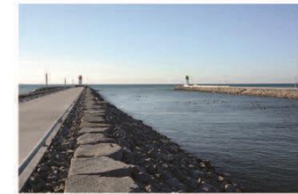
HARBOUR ENTRANCE RECONSTRUCTION CONNECTS THE COMMUNITY WITH THE LAKE
