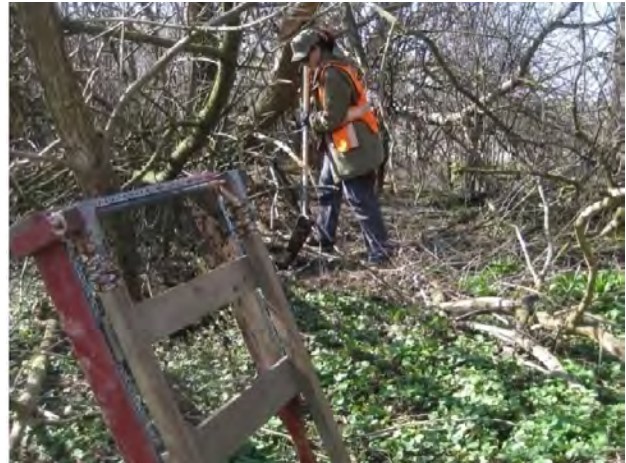
Photo 47: View south southeast. Test pitted dense hedge row.
