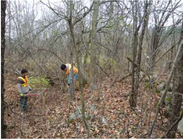
Photo 109: Survey Unit T3-k—View SSE along trunk sewer ROW. Test pit survey of area except wet areas.
