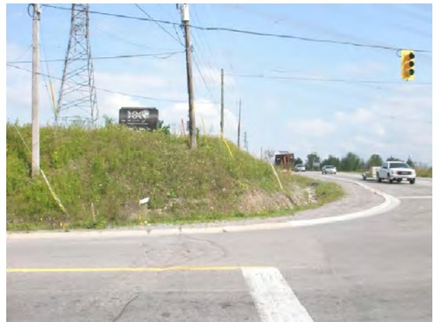
Photo 164: Survey Unit Rossland-g—View NNW at intersection of Brock and Rossland Roads. ROW area disturbed—no potential.
