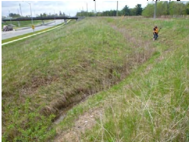
Photo 144: Survey Unit Brock-h—View SSE along Brock Road. Disturbed ROW on west side with built slope and ditch—no potential.
