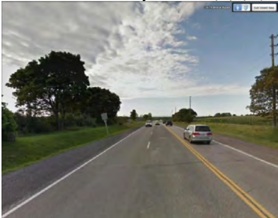
Photo 201: Survey Unit T4-c—View SSW along Brock Road. Disturbed ROW—no potential, Google Earth™.
