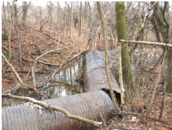
Photo 81: View west southwest. Low and wet area—no potential
