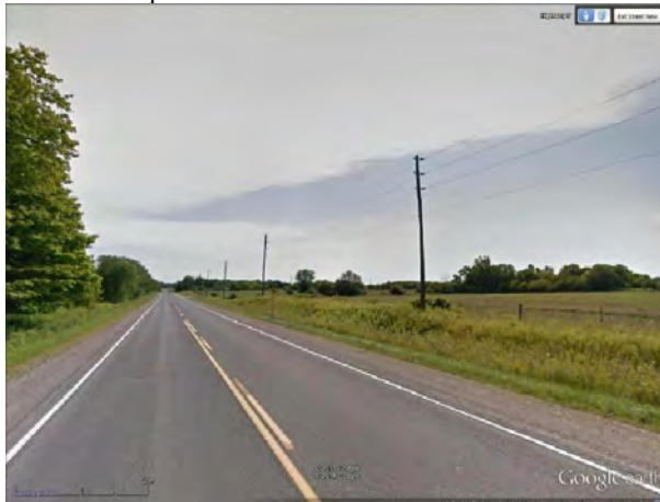
Photo 213: Survey Unit T3-a—View east along Highway 7. ROW disturbed on south side—no pot'.
