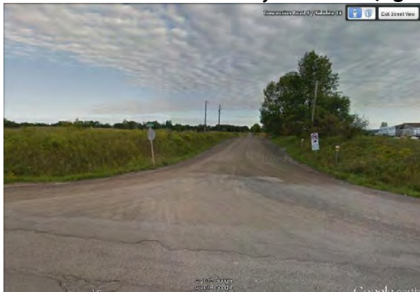
Photo 215: Survey Unit ST4-a—View north along 16 Sideline. ROW disturbed—no potential.
