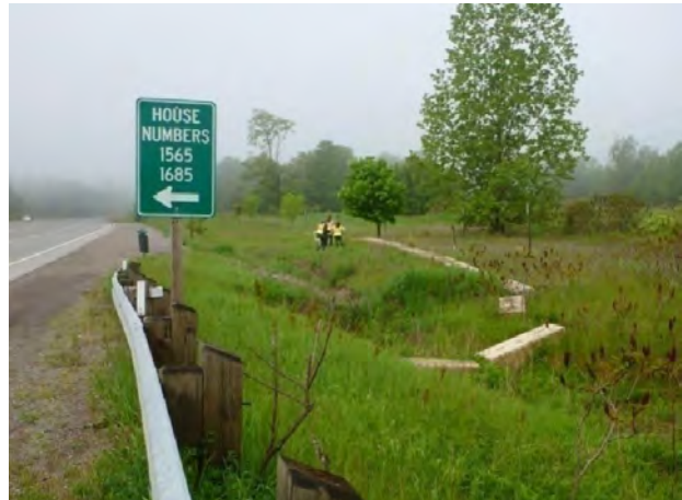
Photo 142: Survey Unit T4-h—View WSW along Taunton Rd. Steep slope on west side—no potential.
