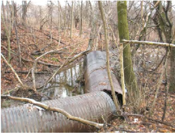
Photo 81: Survey Unit 22 Sideline-d—View WSW along 22 Sideline. Low and wet area—no potential.
