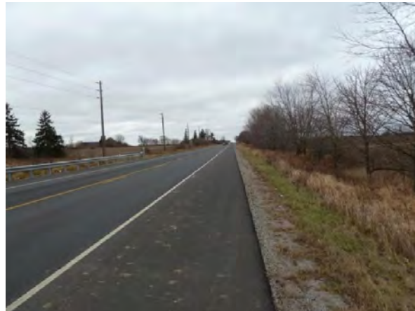
Photo 205: Survey Unit WM2-a— View SW along Highway 7. Disturbed ROW on north side with fill slope and ditch—no potential.
