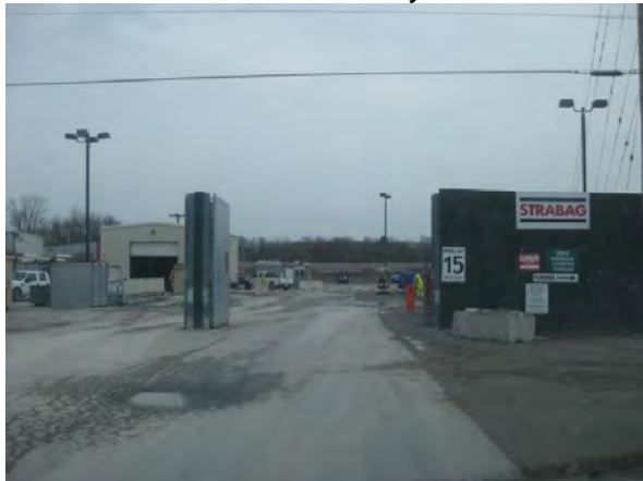
Photo 204: Survey Unit Whitevale-a—View east along new Whitevale Road ROW. Disturbed ROW due to new trunk construction—no potential
