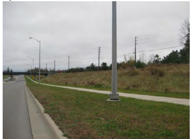
Photo 145: Survey Unit Brock-h—View NNW along Brock Road. Disturbed ROW on east side with utilities, sidewalk and built slope—no potential.
