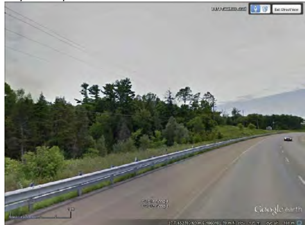
Photo 219: Survey Unit Taunton-j—View SW along Taunton Road. Steep slope on south side—no pot'l. Google Earth™.
