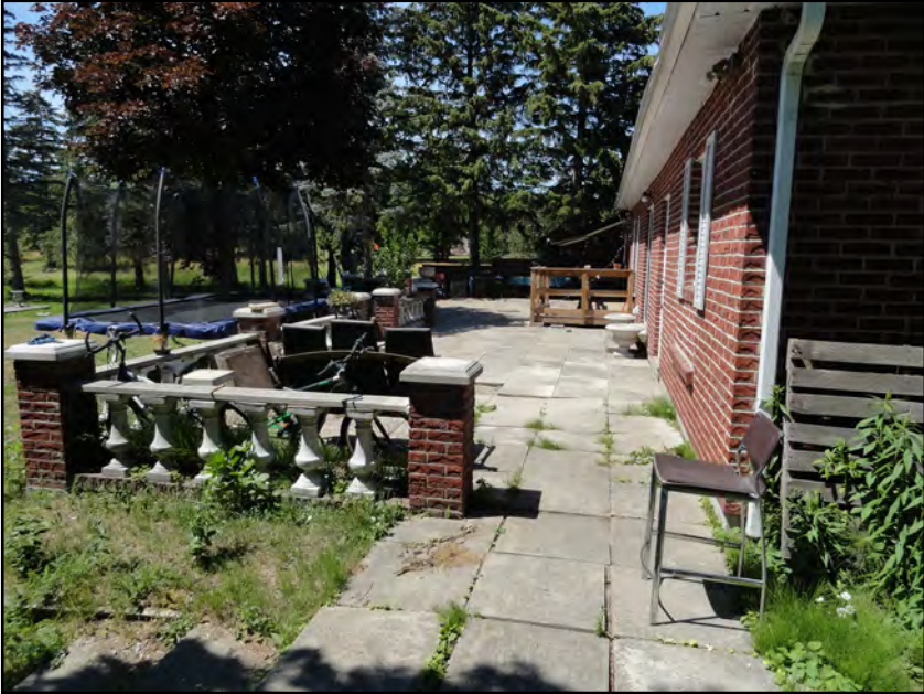
Photograph 5. Attached concrete patio at back of house
