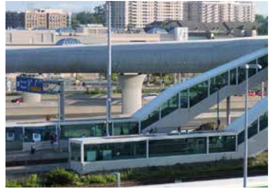
Pedestrian bridge connecting a mobility hub with the City Centre
