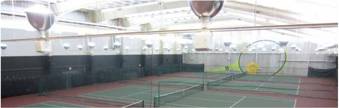
LED lighting retrofit at tennis courts
