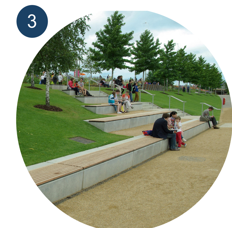
3 TERRACED SEATWALL SEATING W/ SODDED BERM
