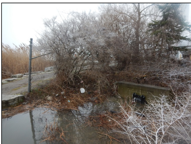
Photo 9: Sloped and wet area at boat launch, note disturbance, facing northwest
