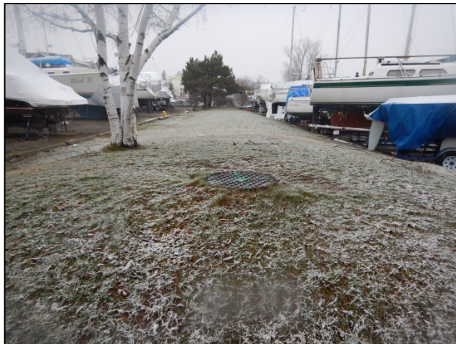
Photo 6: Underground water utilities in landscaped area, facing northwest
