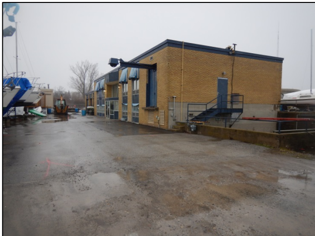
Photo 5: Building footprint disturbance at 591 Liverpool Road, facing northeast
