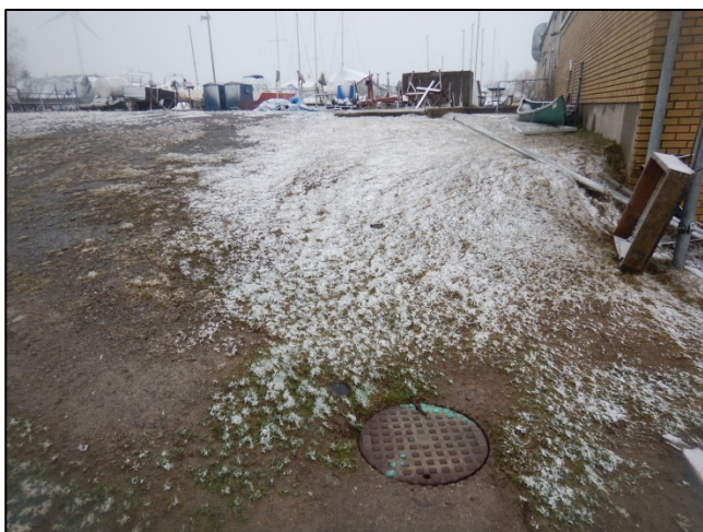
Photo 7: Underground water utilities adjacent to building and parking area, facing south
