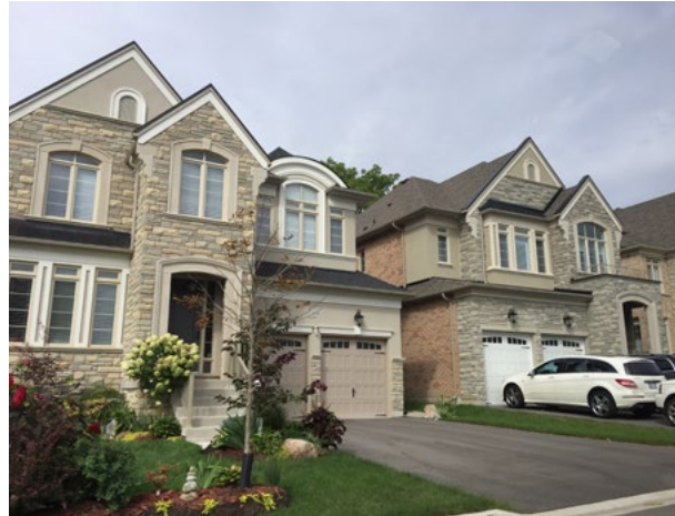
Figure 20: The driveway width is no wider than the garage.
