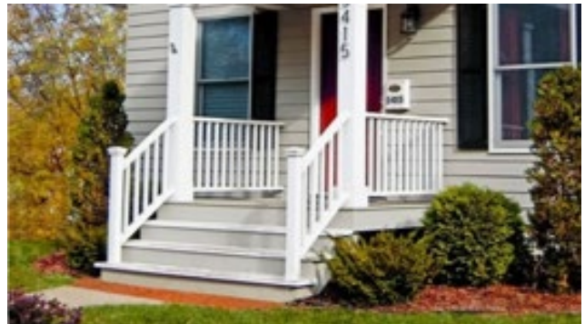
Figure 8: Front entrance with 6 steps or less.
