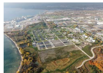
Pickering Nuclear Generation Station, Lake Ontario
