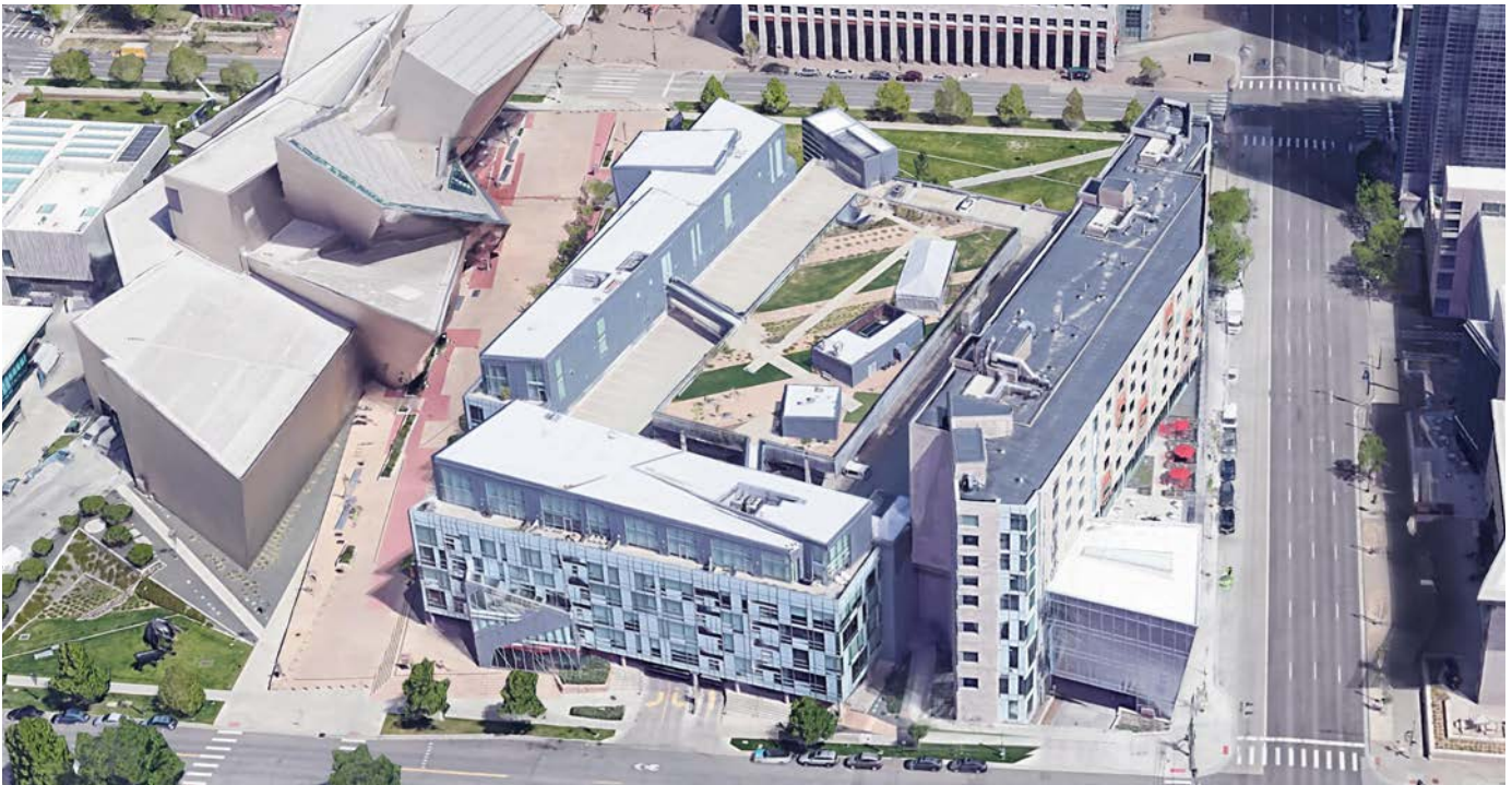
Figure 25. Denver Museum Residence, a 'Texas Doughnut' featuring buildings wrapped around interior parking structure, Denver, USA (photo credits: Google Earth)
