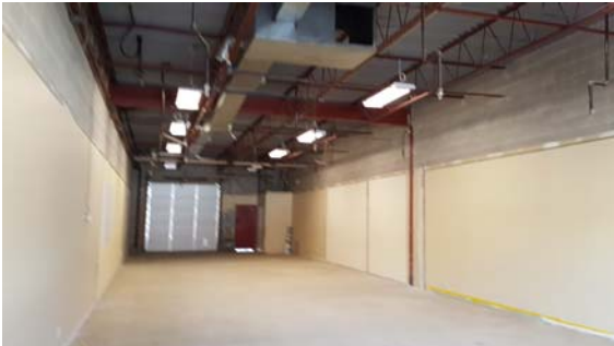
P22 - View of vacant unit in #611 Kingston Road
