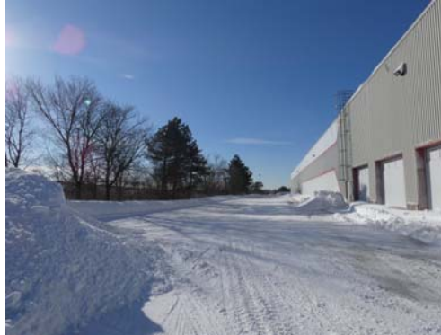
P2 - East elevation of the Site, close to #699 Kingston Road
