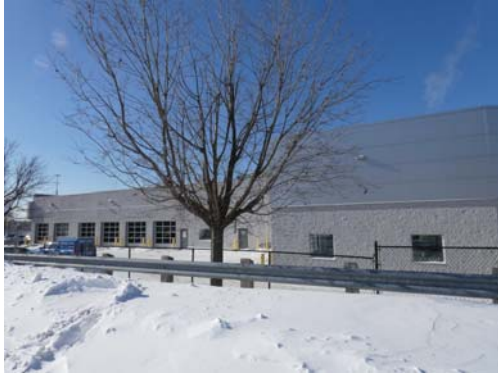
P43 - Neighboring property of the Site to the south
