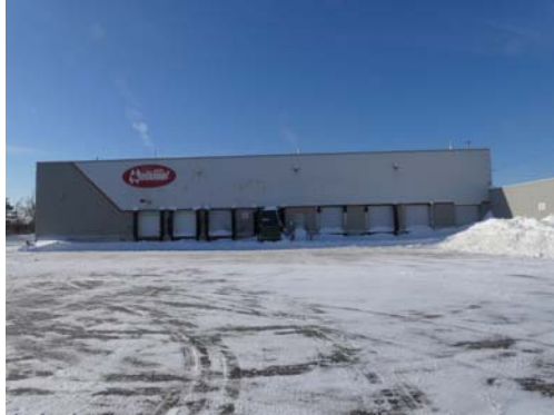
P1 - Front view of #699 Kingston Road
