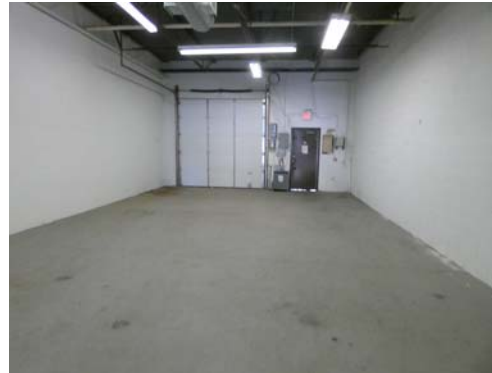
P20 - View of the rear portion of vacant unit in #607 Kingston Road
