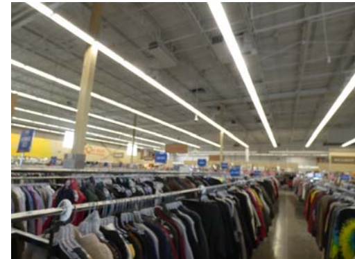
P12 - Partial view of the store on #645-647 Kingston Road
