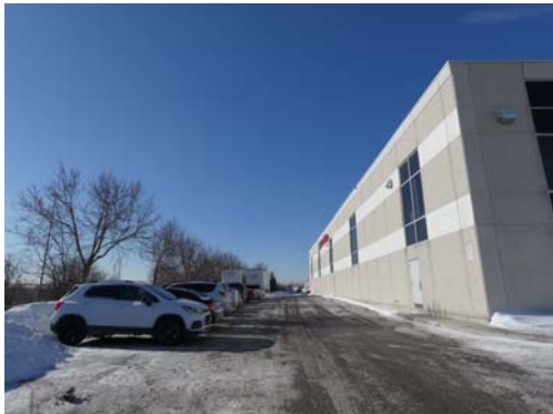
P10 - East elevation of the Site, close to #645-647 Kingston Road
