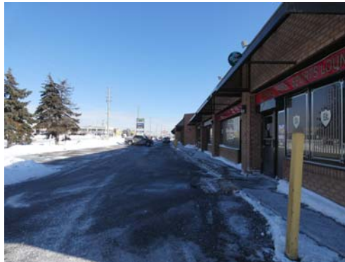
P17 - West elevation of the Site, close to #603-643 Kingston Road
