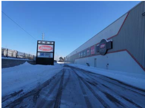
P4 - West elevation of the Site, close to #699 Kingston Road
