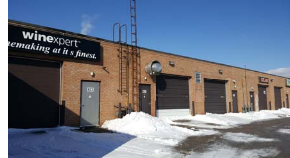
P15 - Partial view of #603-643 Kingston Road
