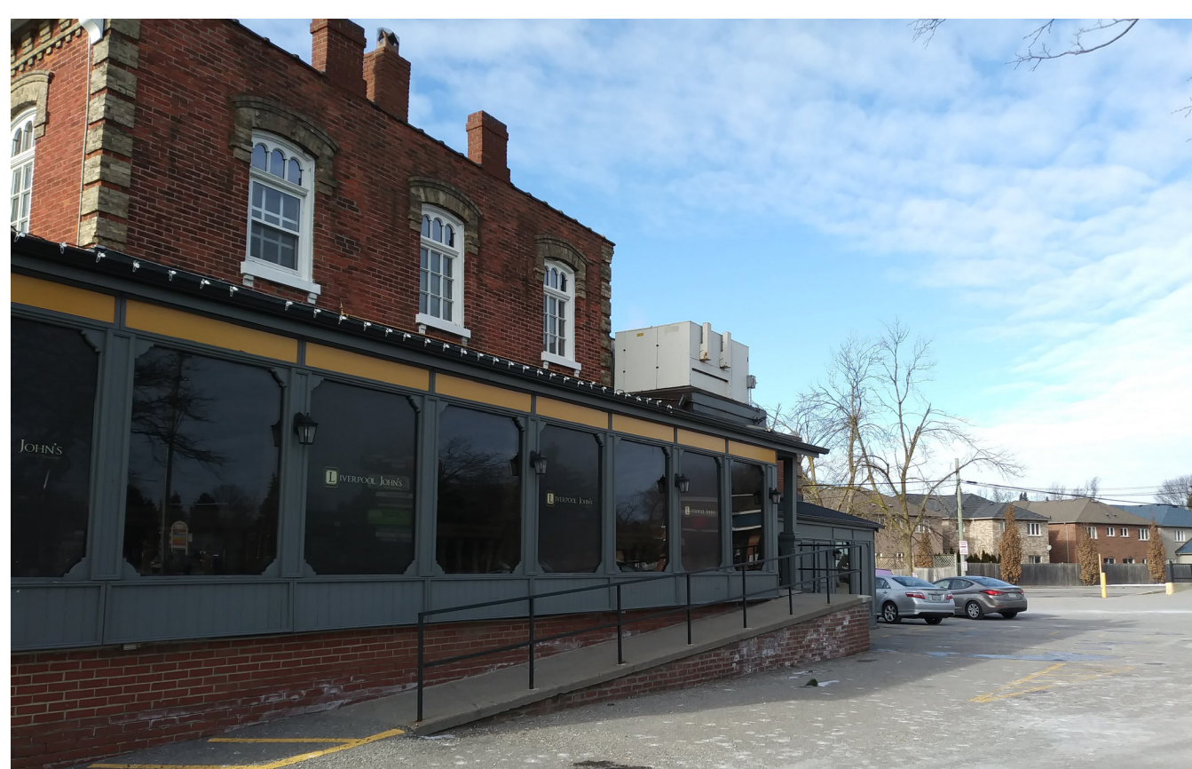
Old Liverpool House facing Liverpool Road
