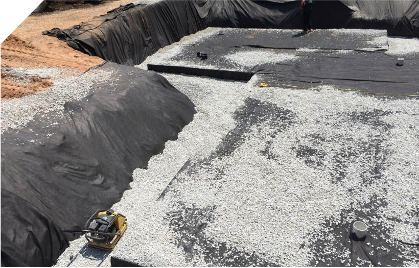
Correctly Backfilled
