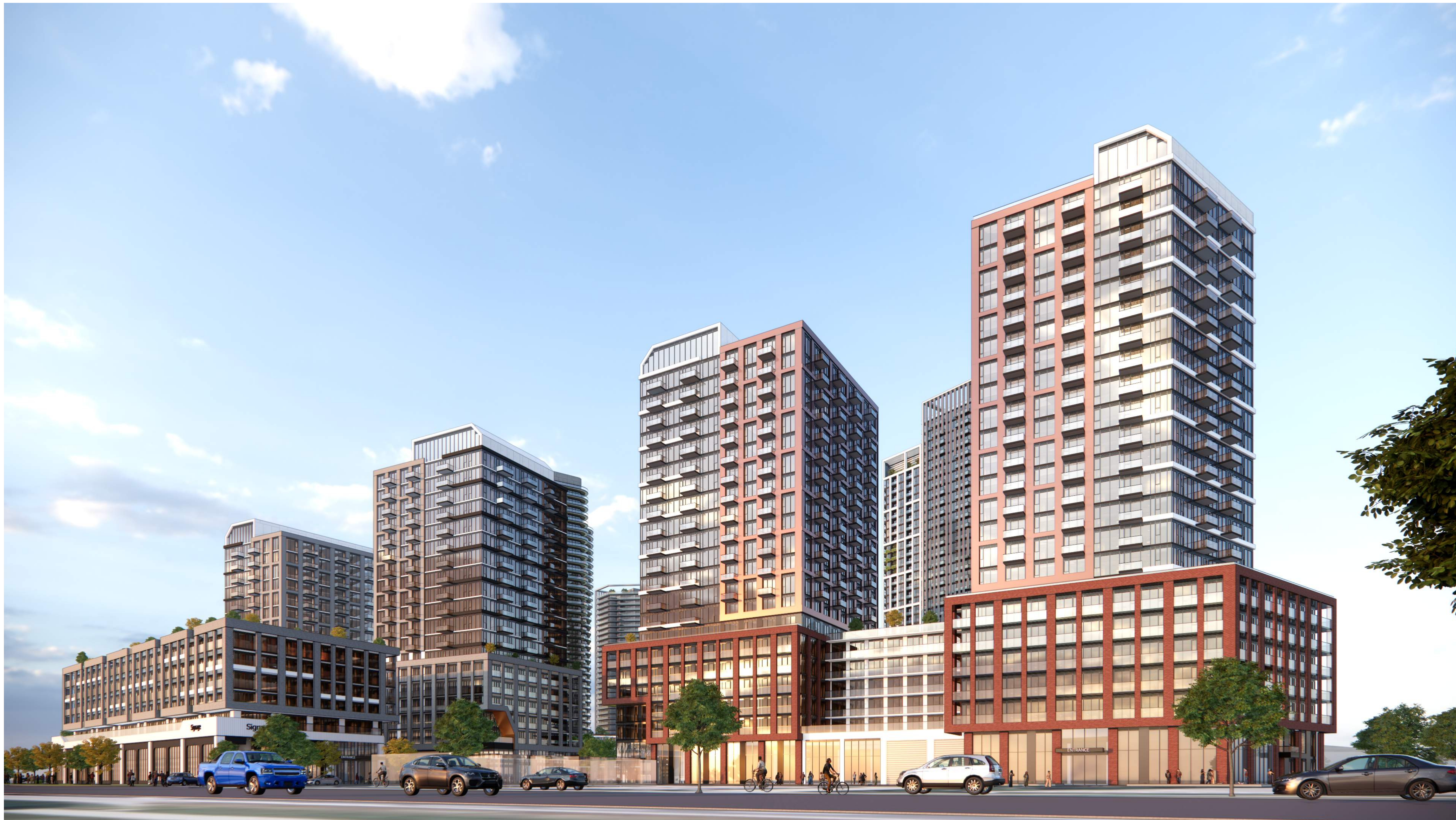
VIEW FROM KINGSTON ROAD LOOKING SOUTHEAST
