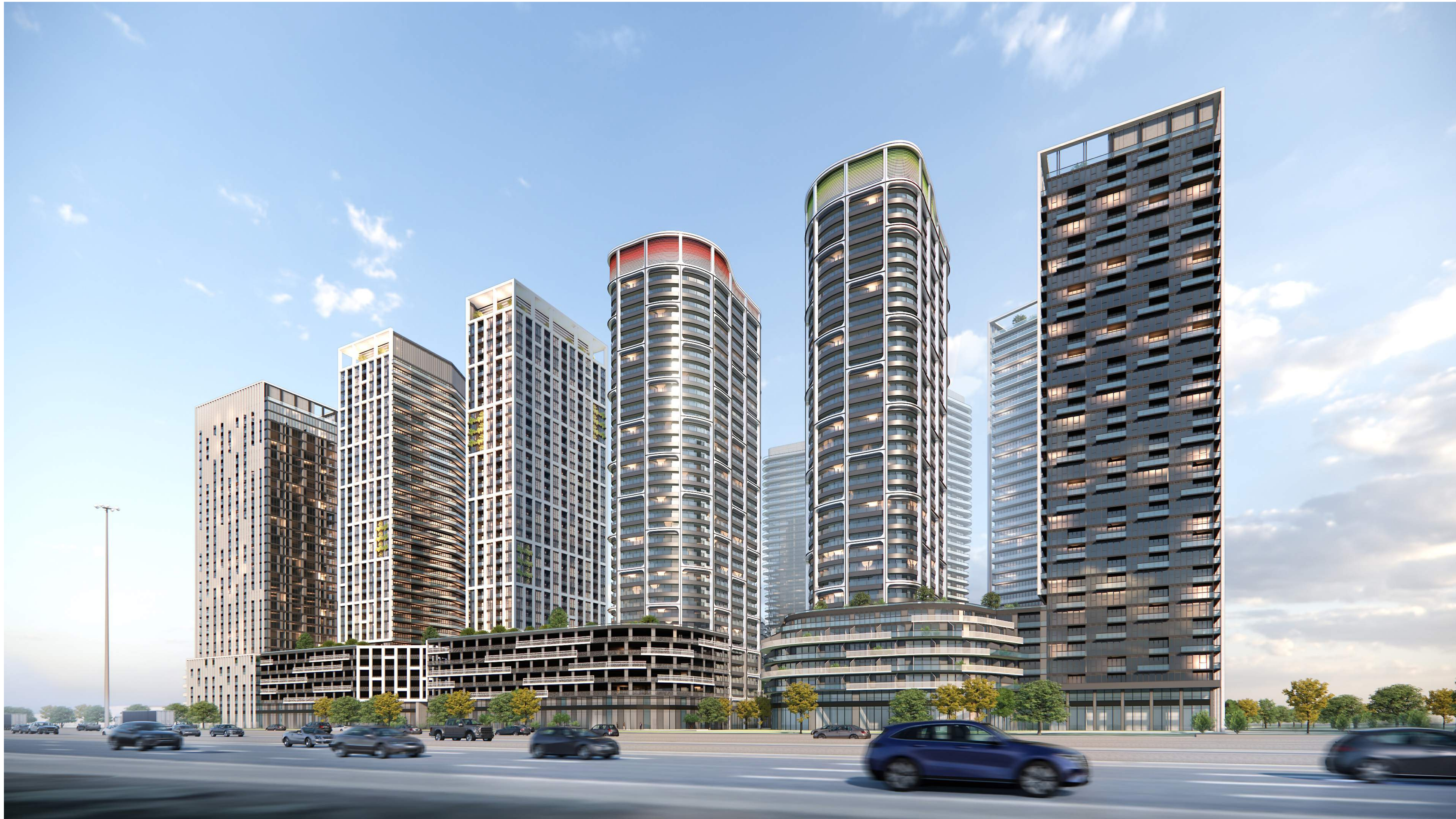
VIEW FROM THE KING'S HIGHWAY NO.401 LOOKING NORTH
