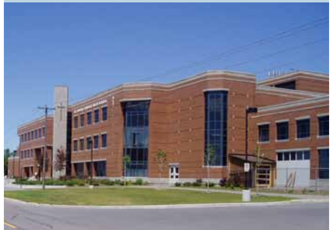
School reinforcing the road edge
