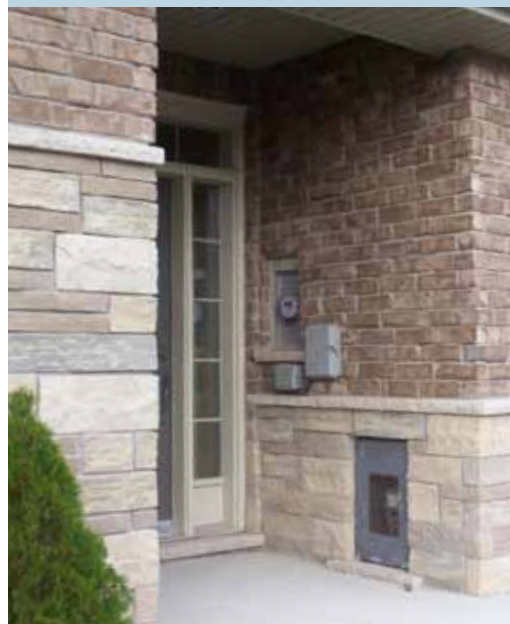
Utility meters should be recessed and hidden from view
