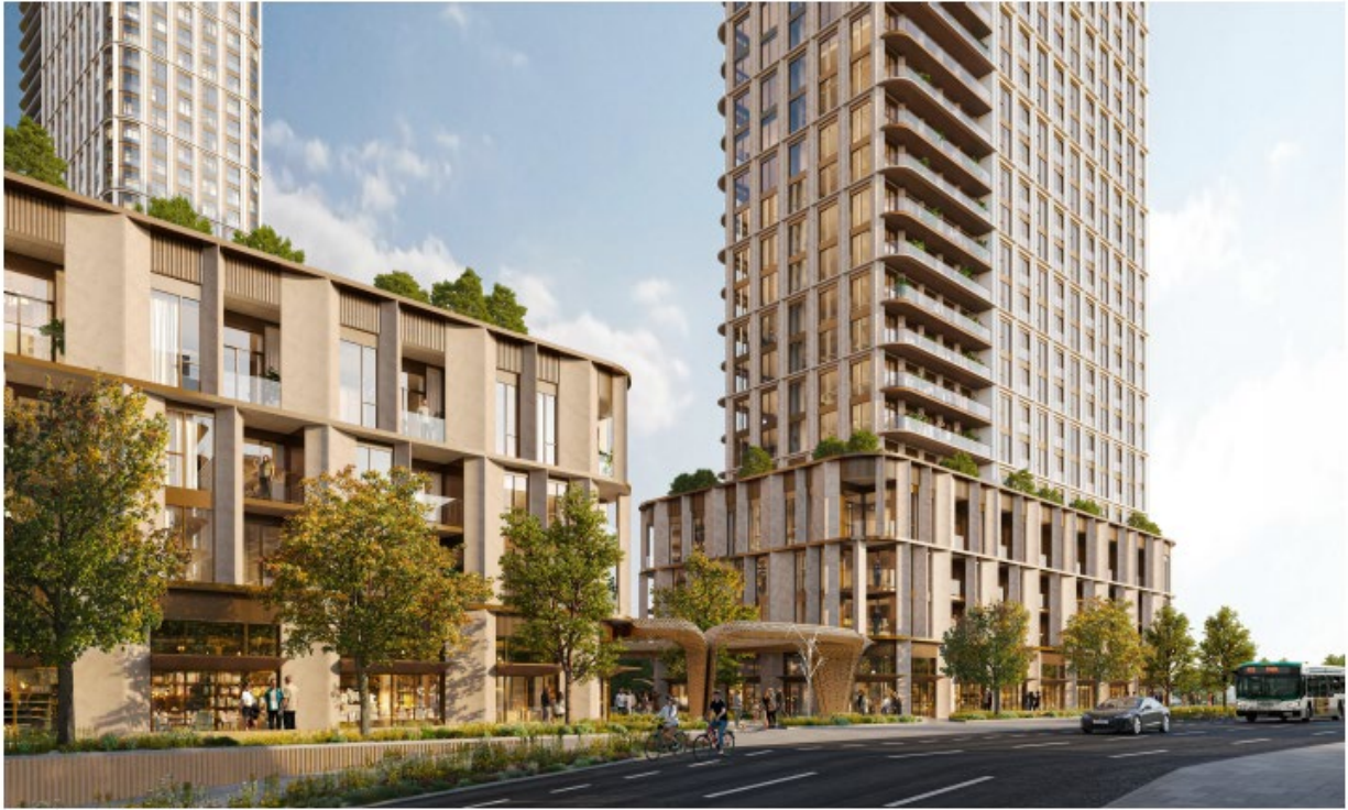
2 Street View From On-Site Public Road Looking Southwest To Gateway
