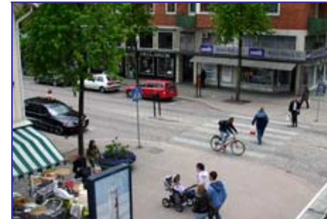
Expanded sidewalks at intersections create safe and convenient access for all pedestrians
