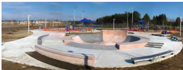
Figure 21. Twelve Oaks Skate Spot, Vaughan, ON. Transition-oriented with a 5' deep bowl, a 'pump bump' in the middle for speed and surrounding plaza space
