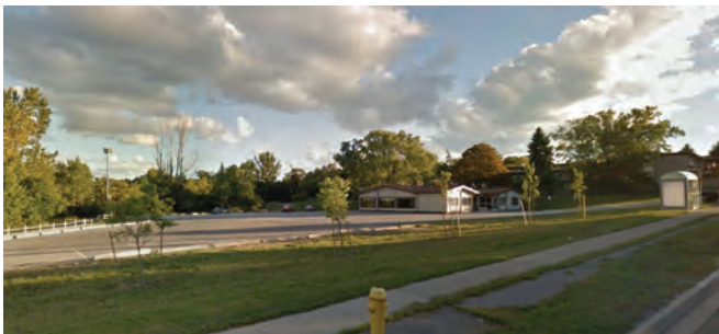
Figure 75. West Shore Community Centre, view from north east
