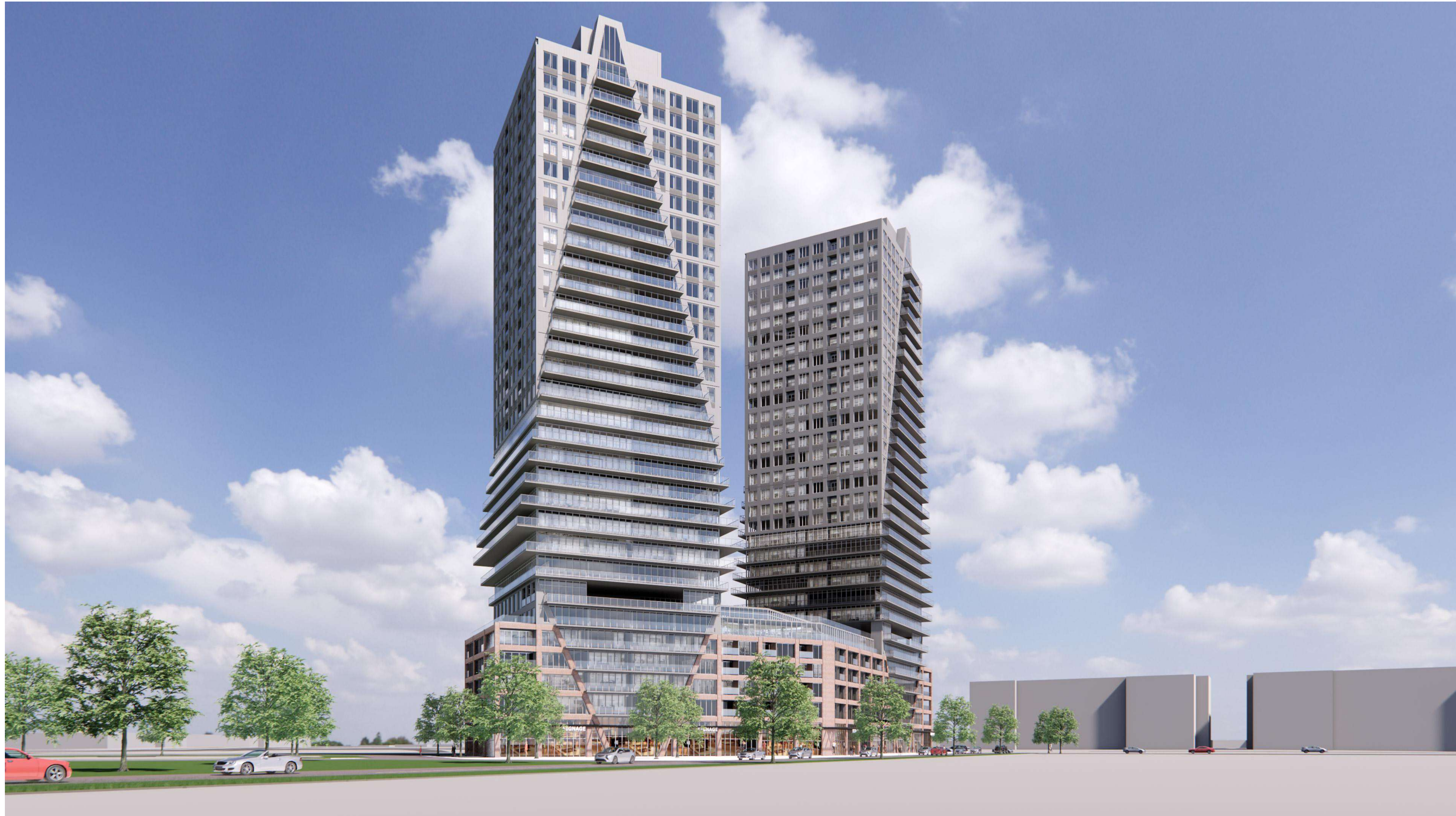
VIEW FROM RIGHT-OF-WAY LOOKING SOUTH
