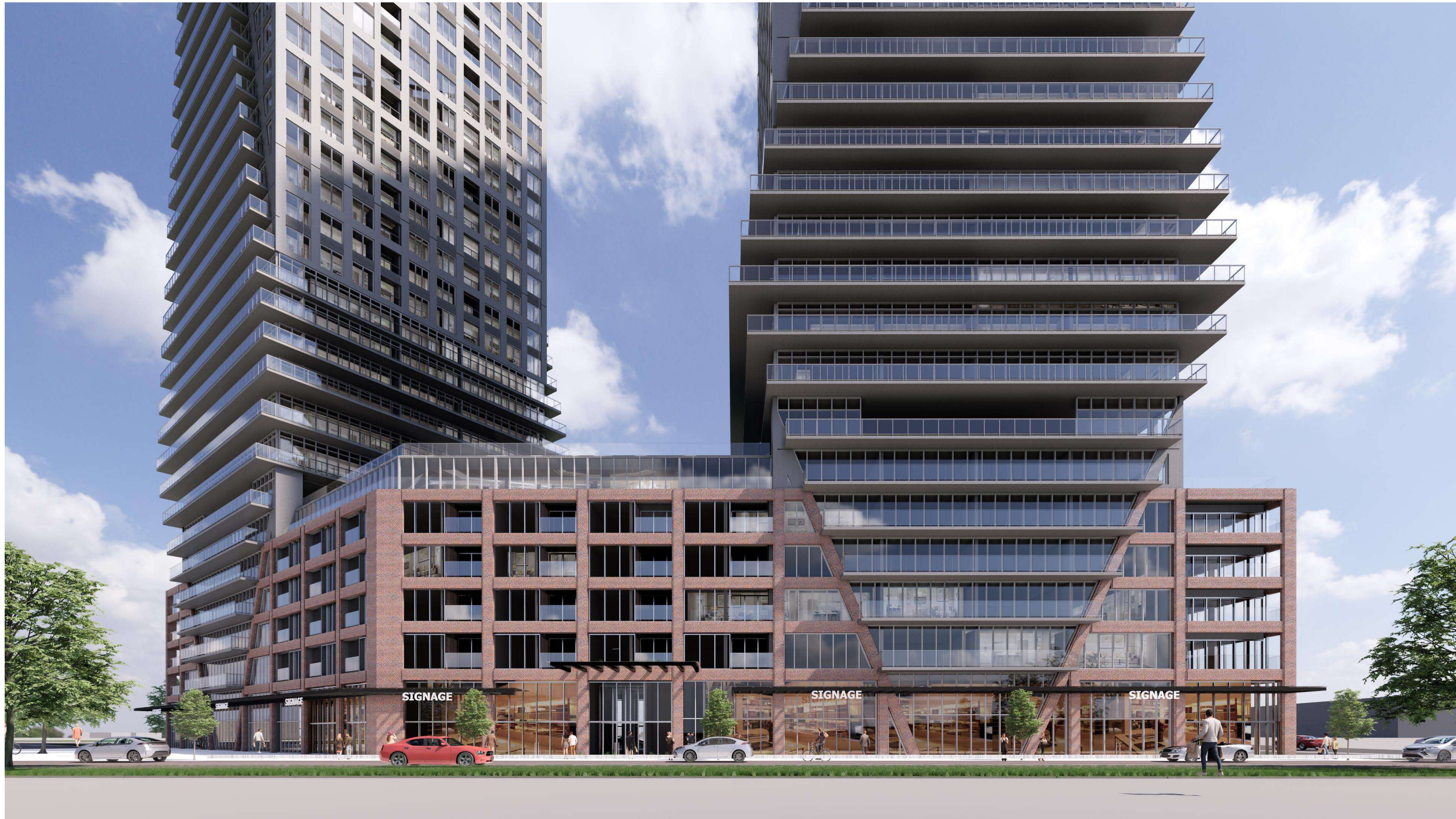
VIEW FROM RIGHT OF WAY LOOKING SOUTH
