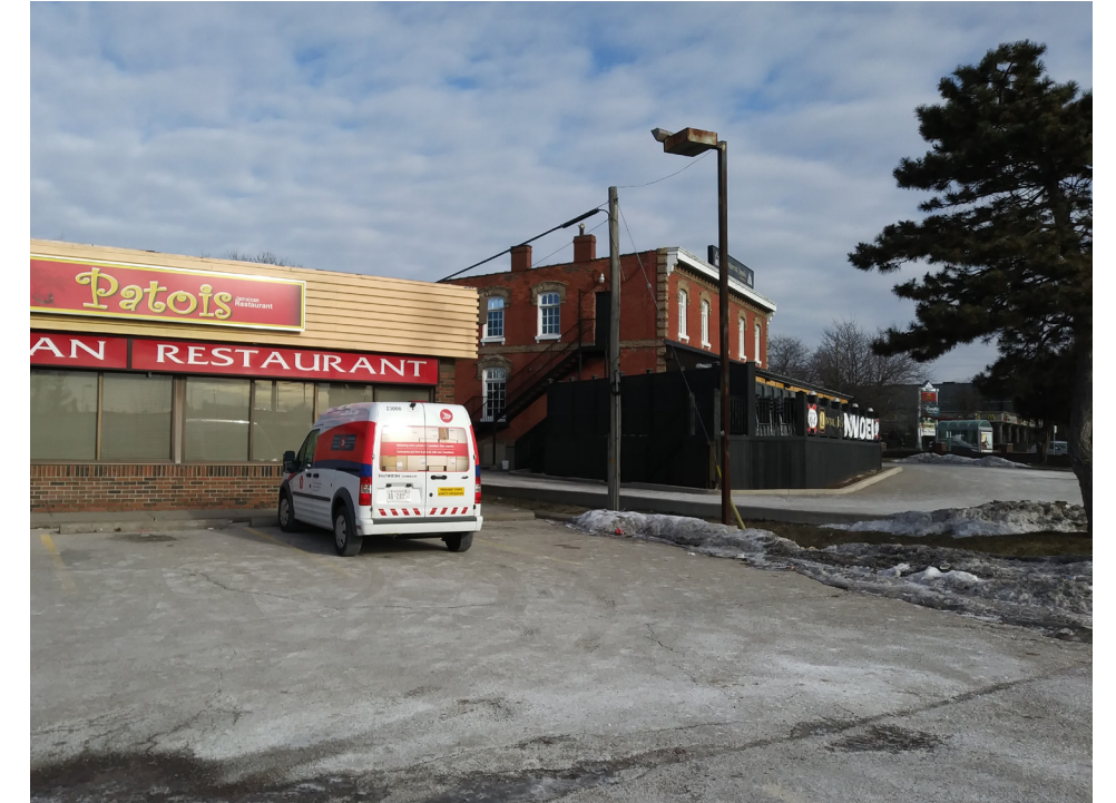
Western edge of site along Kingston Road
