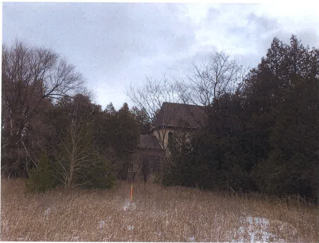
Residential property east of the subject site ( Looking Southeast)
