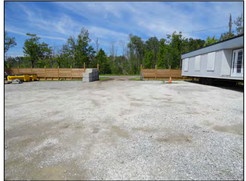
Photograph 10. Westward view towards the front gate and Old Brock Road, of the gravel yard (pad - CVR_4) comprised of approximately 4" of compacted clean crushed and chipped limestone, which was overlain onto the grassed lawn, part of the previous rural residential use
