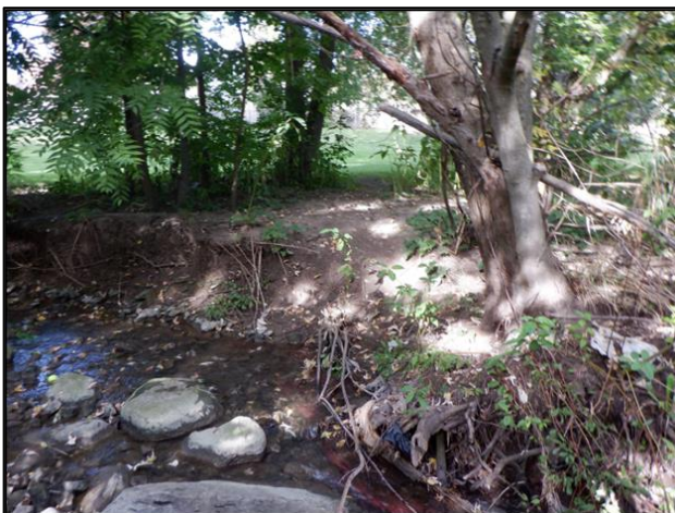
Figure 2-9: Erosion Site #7 – Over Encroachment into the Riparian Corridor Leading to Bank Erosion and a Risk to Parkland.
