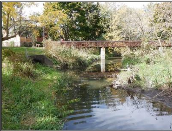
Figure 3-4: Backwater Effects from Beaver Dam Affecting Storm Outfall and Pedestrian Bridge Abutments Upstream.
