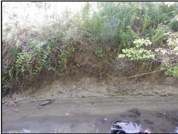
Figure 2-12: Erosion Site #9 – Active Bank Erosion Adjacent to a Multi-Use Trail System
