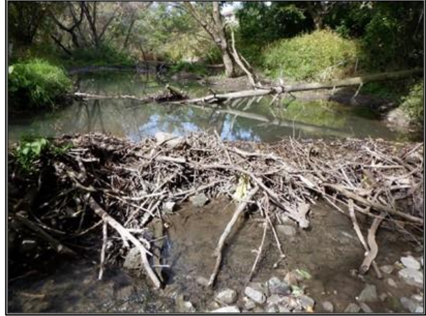
Figure 3-3: Beaver Dam Upstream of Kingston Road Culvert Causing Backwatering of the Reach Upstream.
