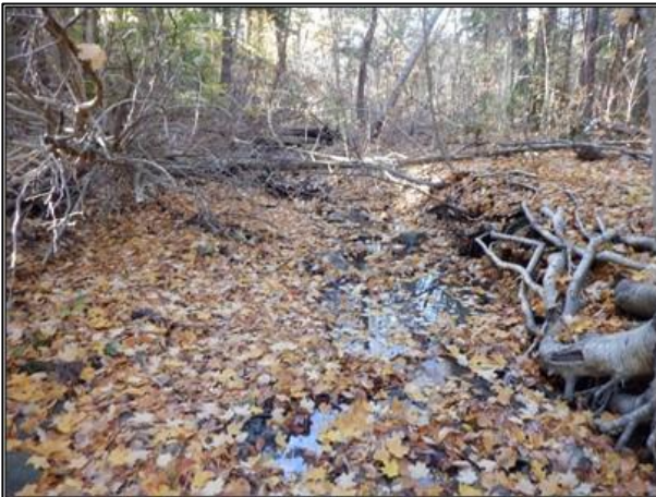
Figure 3-24: Looking Upstream of Channel Where Exposed Tree Roots Through the Banks are Visible.
