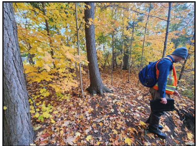
Figure 2-20: Erosion Site #12 – Minimal Offset (<10 m) between Dixie Road Sidewalk and Top of Erosion Scar.
