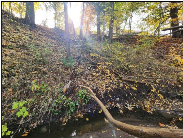
Figure 2-22: Erosion Site #13 – Toe Erosion Creating Risk to Private Property.
