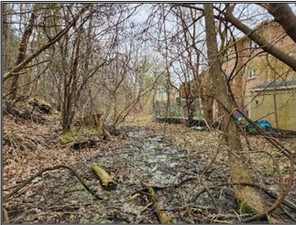
Figure 3-16: Looking Downstream Towards Accumulated Debris.
