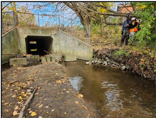
Figure 2-17: Erosion Site #11 – Gabion Baskets Downstream of Dixie Road
