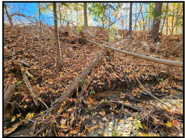
Figure 2-28: Erosion Site #18 – Observed Debris Accumulation and Bank Erosion Adjacent to Finch Avenue.
