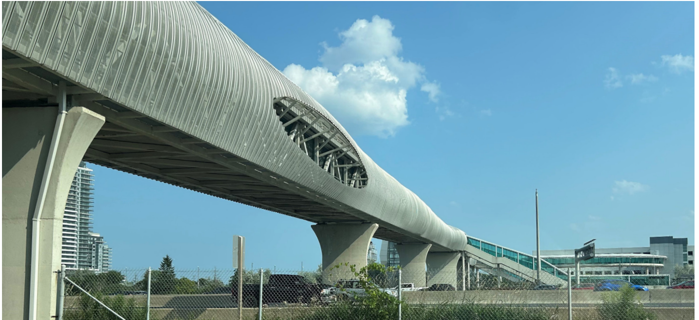
GO Transit bridge over Highway 401, Pickering
