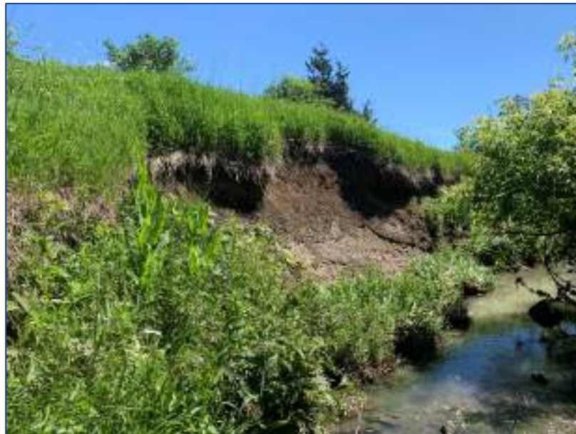
Photo 5. Eroded bank noted on the southeast side of the tributary (June 13, 2022)
