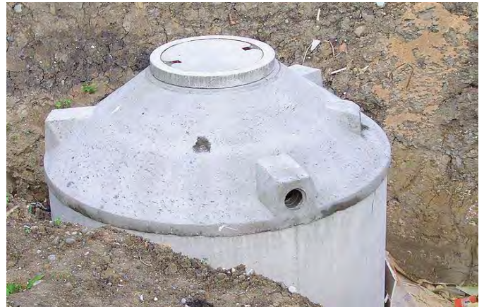
A cistern is an above or below ground water storage system that collects, stores and distributes run-off water of rain or snow from roofs.
