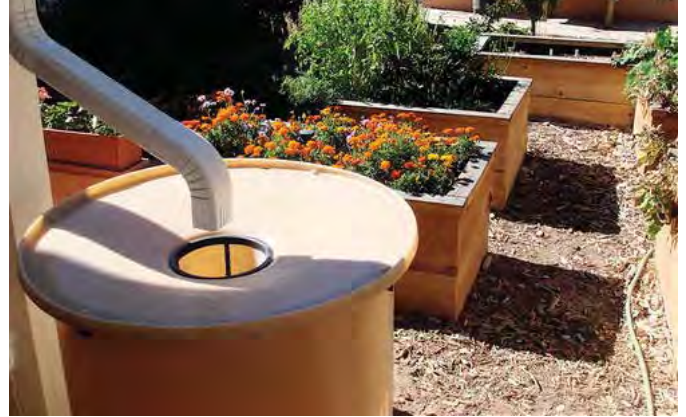
Rain barrels are storage tanks for temporarily holding stormwater. A house can have more than one rain barrel, and barrels vary in size and features.
