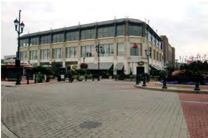
Light coloured pavement reduces solar heat absorption.
