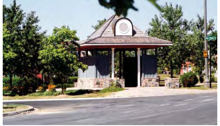
Community features such as a central mailbox and transit shelter are located on the edge of the neighbourhood park.
