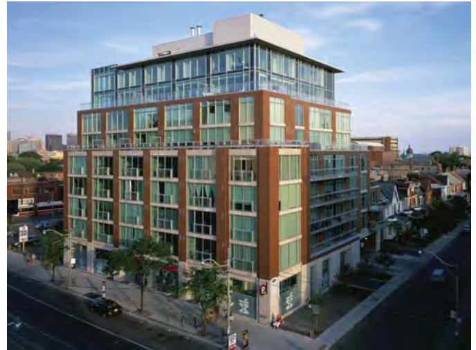
9-storey mixed use building with stepbacks at the street edge, and stepping down towards the residential neighbourhood.
