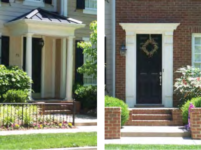
Articulated front entry elements include front steps, roofs, variation in colour and materials.
