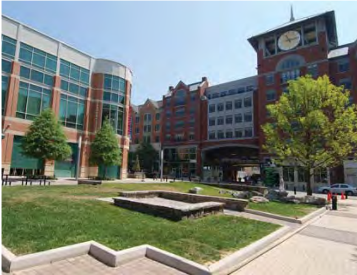
Multi-storey building is massed around a central open space.
