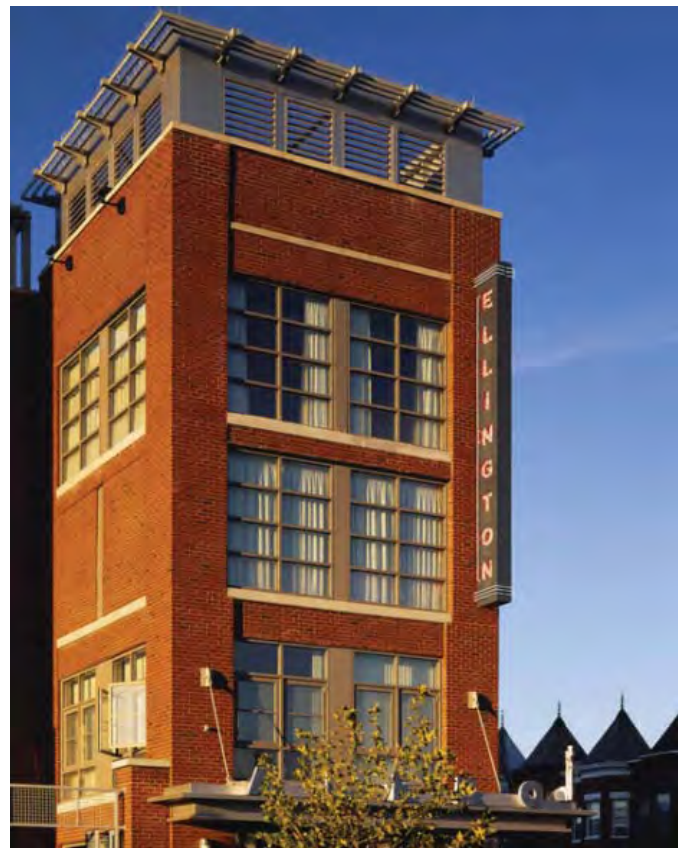
Roof-top mechanical equipment is screened from public view.
