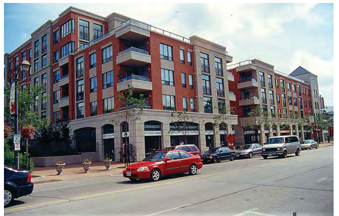
6-storey mixed-use building steps down to 4-storeys along the street edge. The floor above the fourth floor can accommodate a shared amenity area, such as an outdoor roof, for residents.
