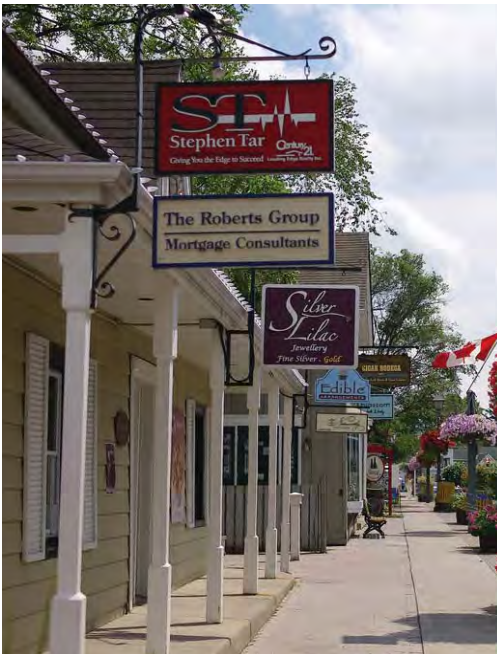
Hanging signs encroach over the streetline and extend into the pedestrian realm.
