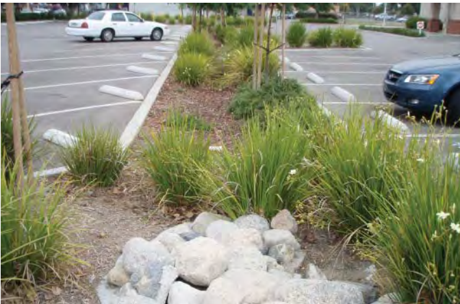
Bioswales slow water run-off, and clean and filter water, and can be integrated into parking lot designs.
