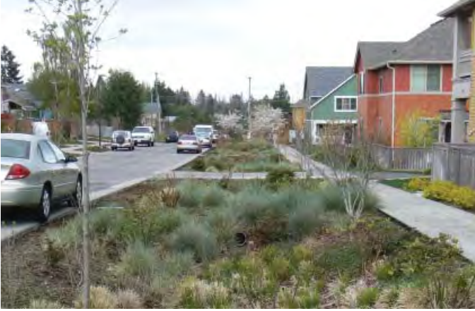
Bioswales can be integrated along roads, planted with long-rooted native plants that absorb large quantities of water.
