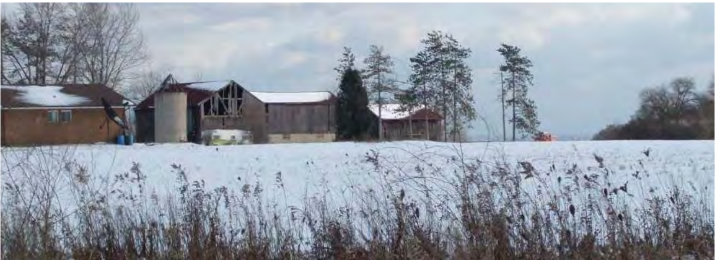
John Tool House, 1.5 storey stone barn
