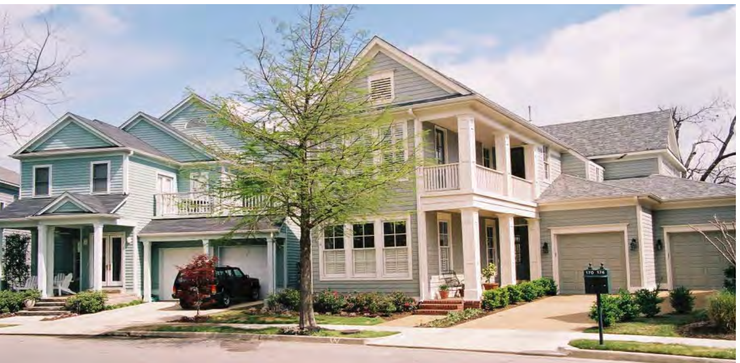
The width of driveways should be minimized and should taper where it meets the sidewalk.
