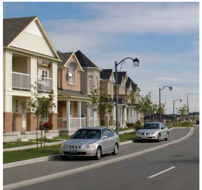
In residential areas, on-street parking bays should be provided on collector and arterial roads for visitor parking.
