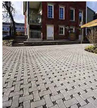
Permeable pavers can be used in pedestrian areas or for vehicular applications.
