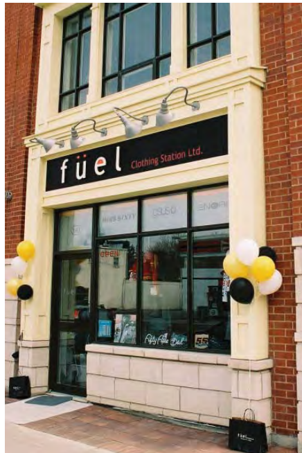
Lighting above signage is directed at the sign and complements the design of the building.
