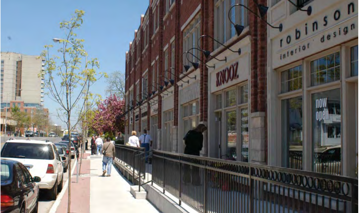
A consistent building wall helps define the streetscape and creates a sense of enclosure.
