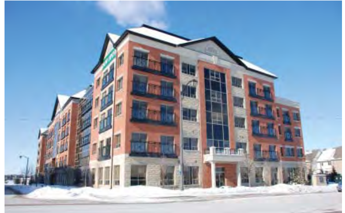
5-storey residential building frames the street edge and addresses both streets.
