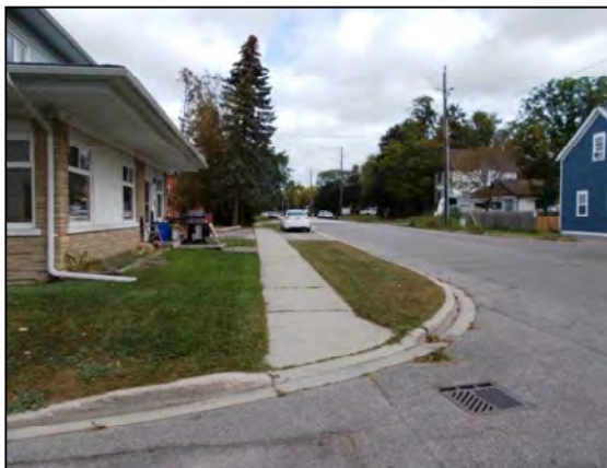
Photograph 55: Facing north, intensive testing required on manicured lawn.
