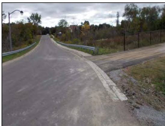
Photograph 27: Facing southeast, intensive testing required on fairly level areas.
