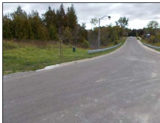
Photograph 28: Facing east, intensive testing required on fairly level areas.
