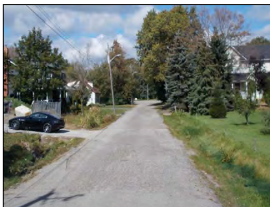
Photograph 99: Facing north, intensive testing required on manicured lawn.
