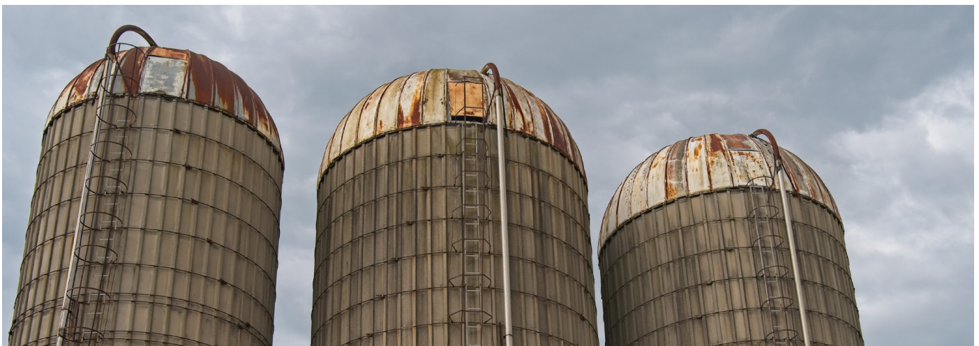
Silos for grain storage
