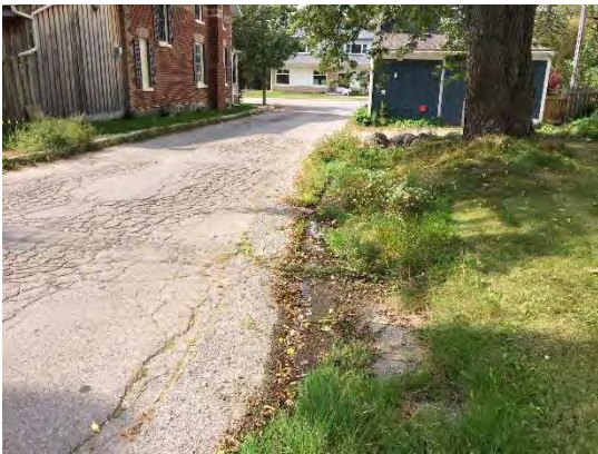
Photo 69 Joseph north side west of Old Brock Road
