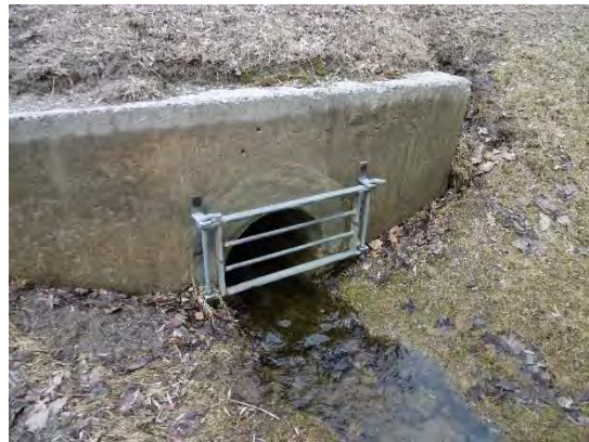
Photo 94 Central Street Outlet (Creek)
