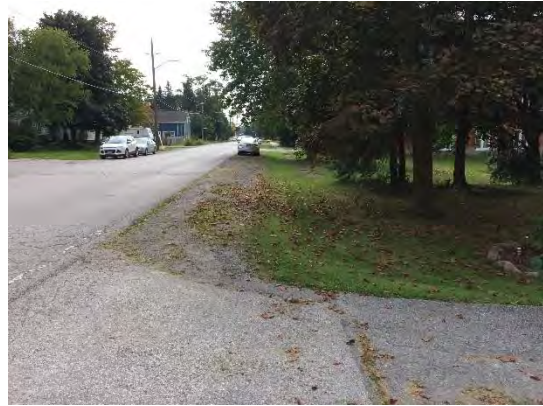
Photo 74 Old Brock Road north of Central
