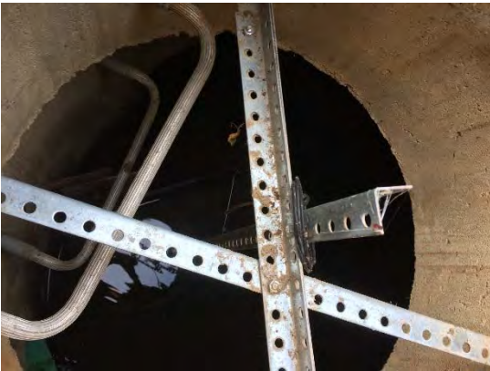
Photo 21 Central Street Control MH
