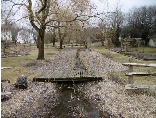
Photo 103 Central Street Outlet (Creek)
