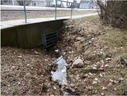
Photo 97 Central Street Outlet (Creek)
