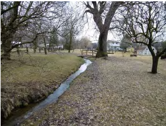
Photo 93 Central Street Outlet (Creek)
