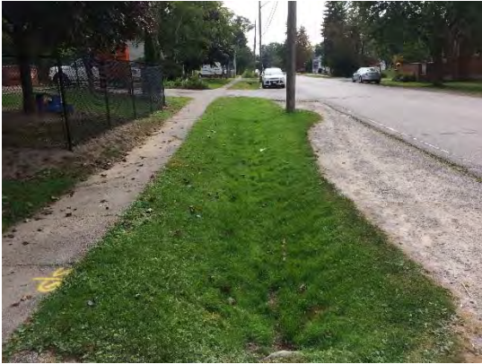
Photo 73 Old Brock Road north of Central
