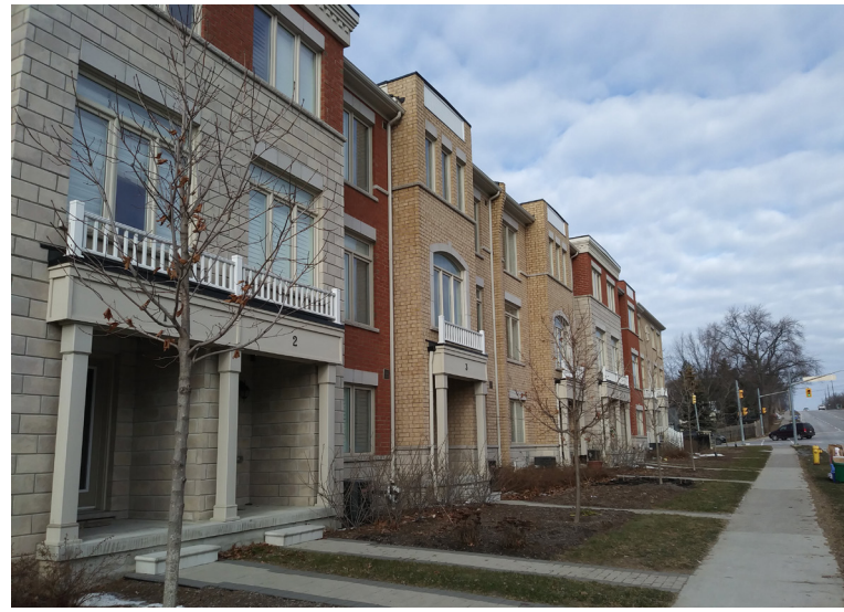
> Three-storey townhomes north of the subject site on Liverpool Road, looking north.
