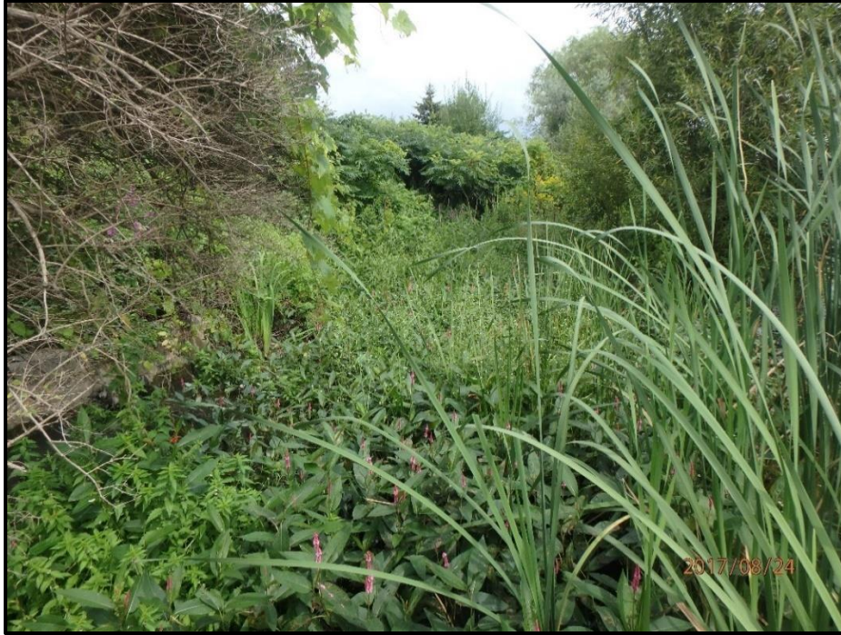
Photograph 2. Water Smartweed Inclusion at Headwall
