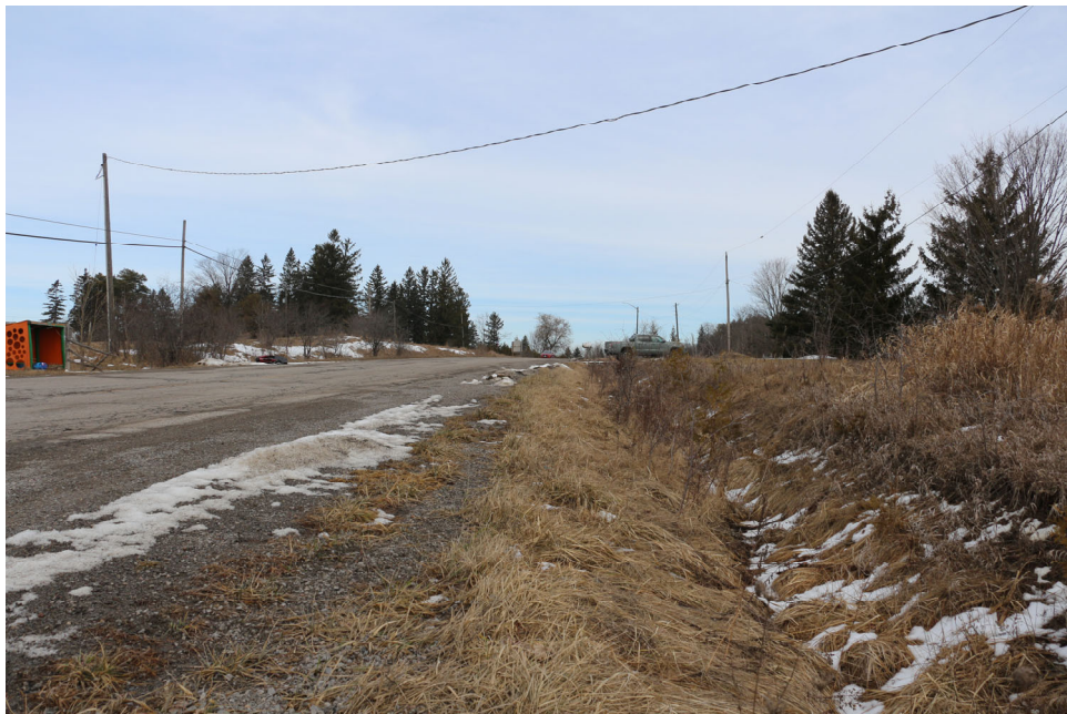
At North Access location looking north (view to the right)
